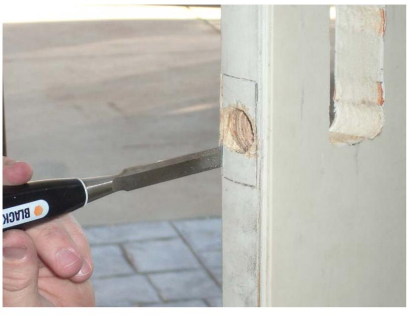
This step may be optional depending on the spacing of your door and the setup of your door jamb. The holes for the latch/deadbolt need to be counter-sunk into the door, if needed mortise the latch/deadbolt into the edge of the door.
