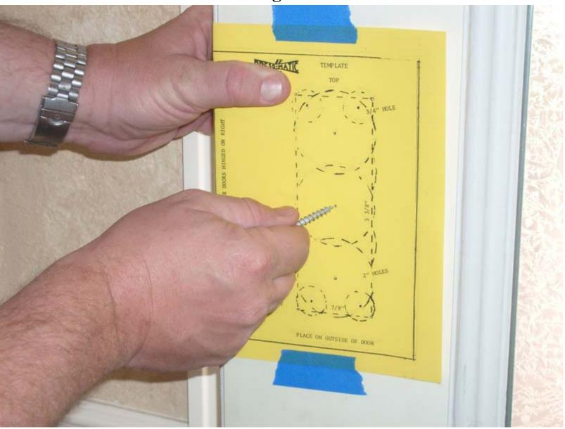
Mark the four corners as well as all the center holes to be drilled out, this can be done using a Scratch-Awl, a nail, or as pictured a screw. Be sure to make the indentations deep enough, else the drill will run out the hole and marr the door. Be cautious with wood doors as they can split or chip.
