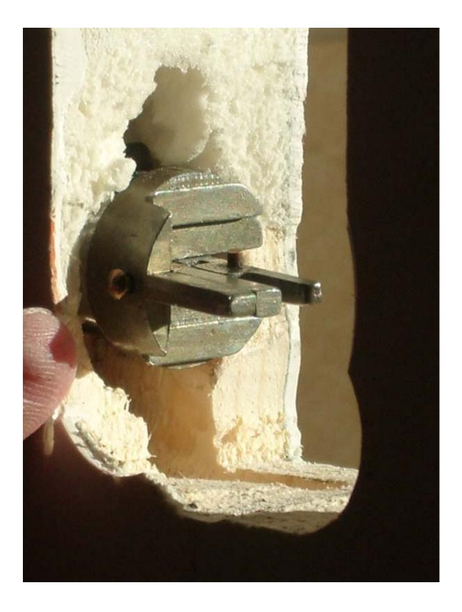
With the brass pin inserted into the deadbolt it will hold the deadbolt in the 'extended' position.
