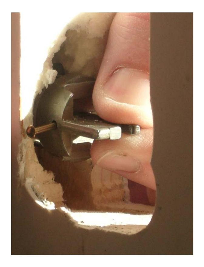
Place the small brass pin into the hole in the deadbolt housing, insert all the way through into the channel on the actuator. This will hold the deadbolt in the 'extended' position and make the insertion of the lock into the door much easier.
