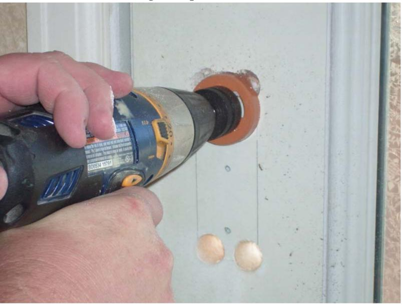
Drill the holes using a hole saw. There are alternative methods of cutting the door, if the door is a solid wood door, the best and most acurate (albeit slowest) method is to use a coping saw. For metal skinned (but hollow) doors a Dremel or similar tool can be used. A Jigsaw or Sawz-all can be used, but be cautious to watch both sides, the blade on the opposite side of the door can track and follow a different path, resulting in a curved cut.
