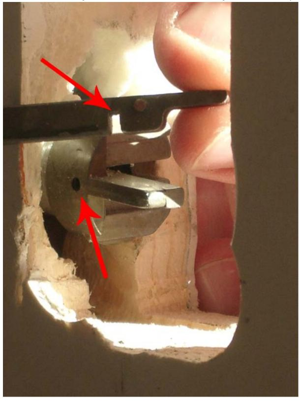
Put the actuator into the deadbolt, the small channel should line up with the hole on the actual deadbolt.
