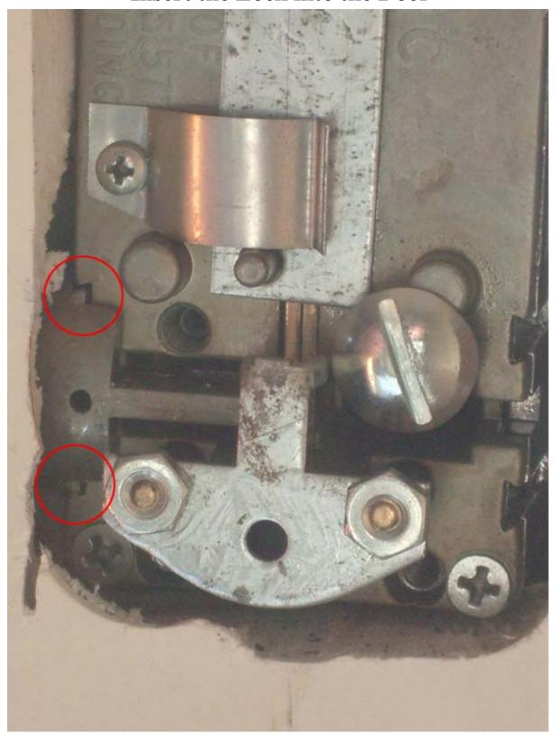
Align the two dovetails and slide the lock body into the door. Reinstall the large headed screw with the long thin spring under it, tighten snugly, be cautious to not overtighten as it can cause binding issues.
