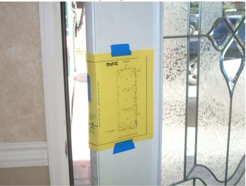
Tape the template to the door securely so it will not move, otherwise the markings for where to drill the holes may be off.
