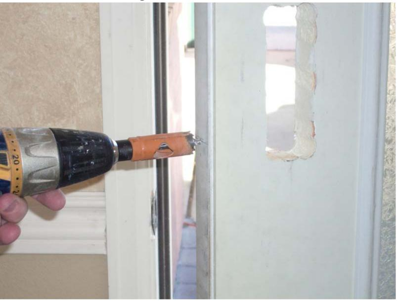
Cut the hole for the latch/bolt. Be careful to drill the hole as level as possible (in relation to the hole cut for the lock), if it is off by much it can cause binding or a 'sticky' lock.
