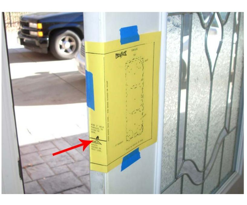
Also be sure to mark the bore for the bolt or latch (Mark on the spot labeled "Locate center on this line")
