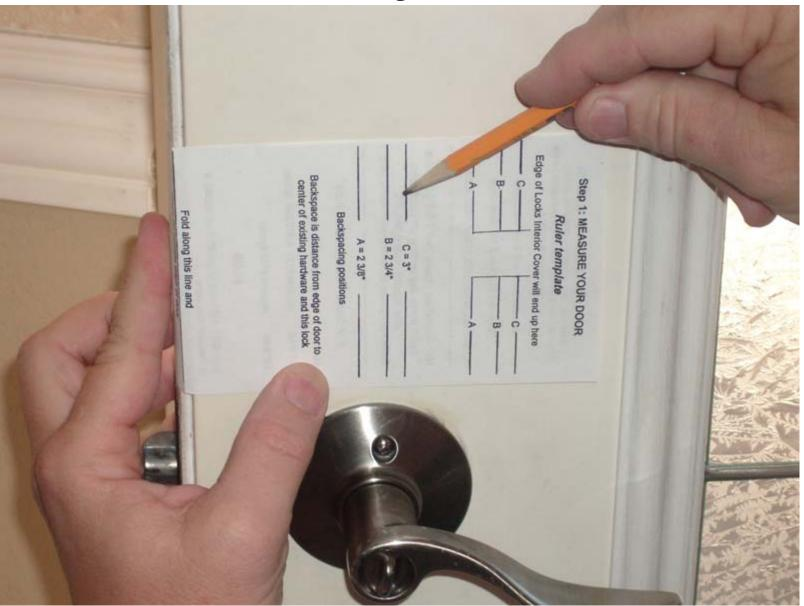
Open up your instructions and remove the template labeled "Step 1: MEASURE YOUR DOOR". Fold along the line and use this template to confirm that the lock has the proper backspacing and will not interfere with existing hardware once installed.
