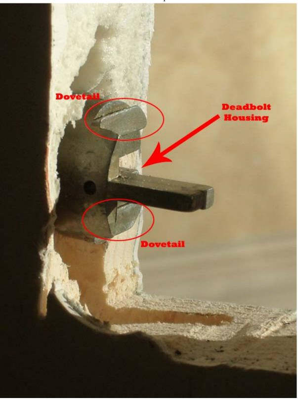
Insert the deadbolt into the door, for a Long-Throw deadbolt model, ensure that the multiplying lever swings fully in the channel made for it. On the edge of the door install the screws but do not tighten them all the way down.
